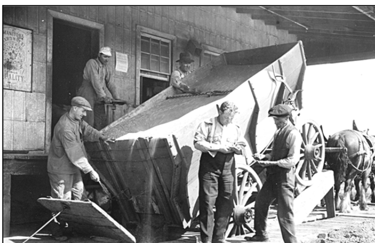
Figure 11: Wagons and Trucks . Two photographs showing grain being dumped into an elevator "pit" by means of a mechanical front-wheel lifting device. From the pit, the grain would be "elevated", using a "circular belt and bucket" drive referred to as a "leg"; and from the top of the elevator the grain could be directed into storage bins, cleaners, or railway boxcars.
