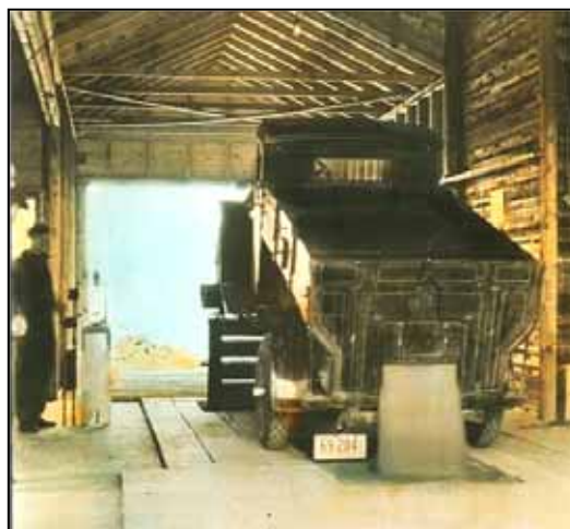
Figure 11: Wagons and Trucks . Two photographs showing grain being dumped into an elevator "pit" by means of a mechanical front-wheel lifting device. From the pit, the grain would be "elevated", using a "circular belt and bucket" drive referred to as a "leg"; and from the top of the elevator the grain could be directed into storage bins, cleaners, or railway boxcars.
